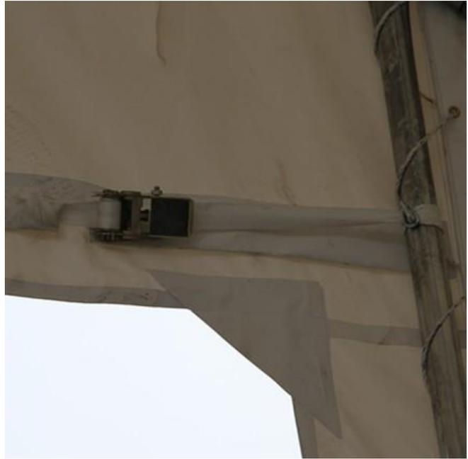
**NOTE: DO NOT LEAVE THE ROOF COVER UNATTACHED UNDER ANY CIRCUMSTANCES** until the final assembly and tightening has been completed. The process is quite easy. But some tightening adjustments will be necessary to produce a flat, tension ed roof cover. Please adjust the roof cover every month.
